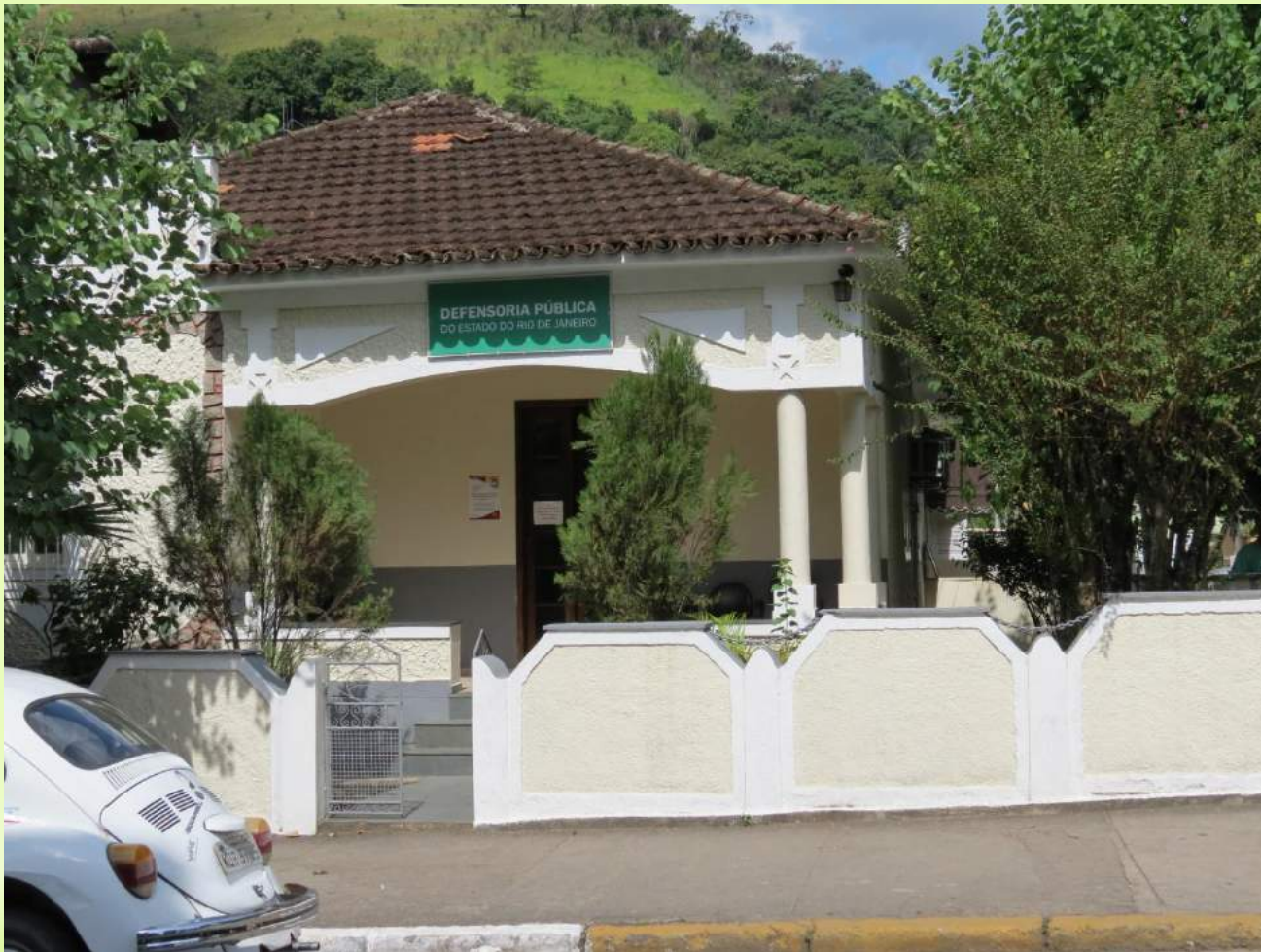
Local branch office of the PDO in the town of Cachoeira de Macacu (Rio de Janeiro State)
